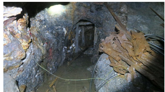
Haulage way (on rails), old Dawson workings as seen in 2023; with rusted-out equipment.
