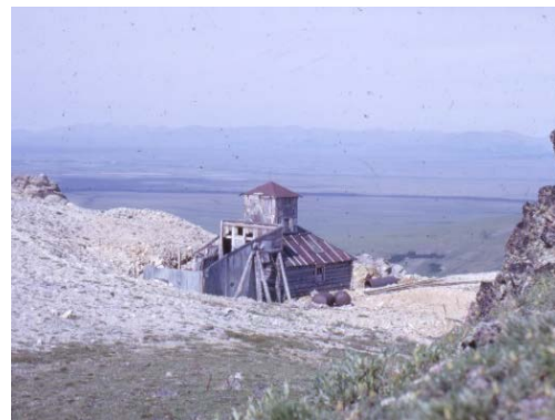
The Omailk lead-zinc-silver mine in 1964, Alaska’s first productive base metal mine, Seward Peninsula (DM&M Geo Report 11).
